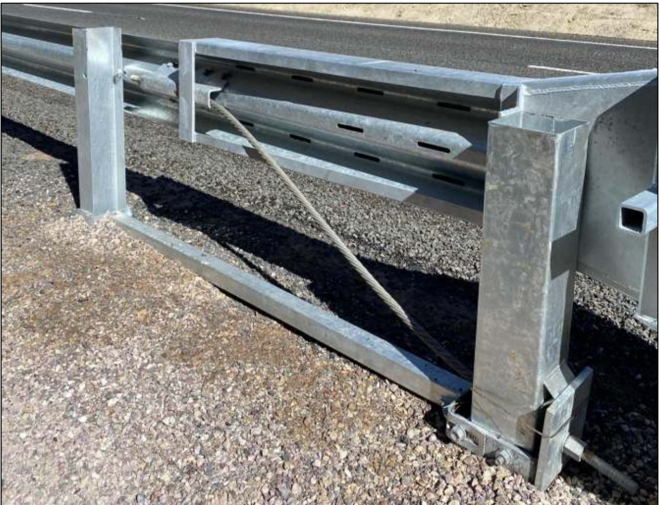
Figure 12: MSKT Anchor Assembly – Rear View
