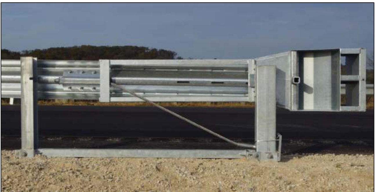
Figure 9: Attachment of Cable Anchor Bracket
