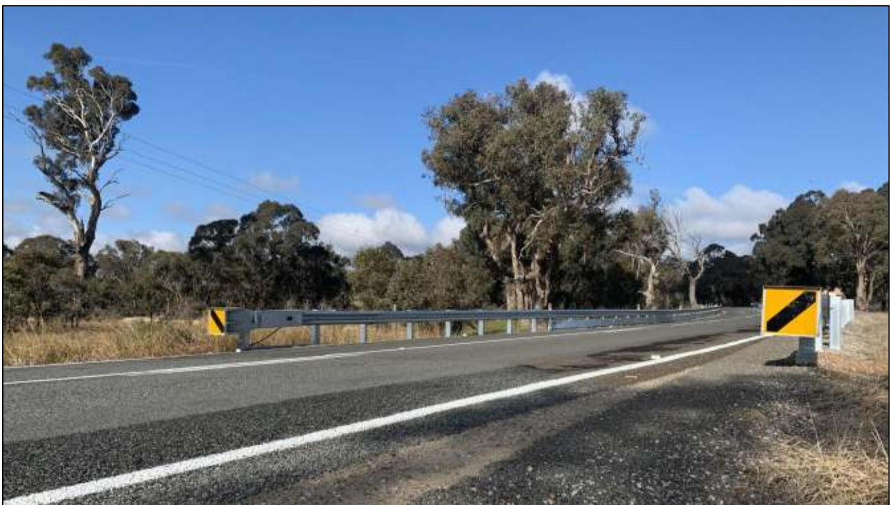
Figure 6: MSKT Rail Lap for Opposing Traffic
