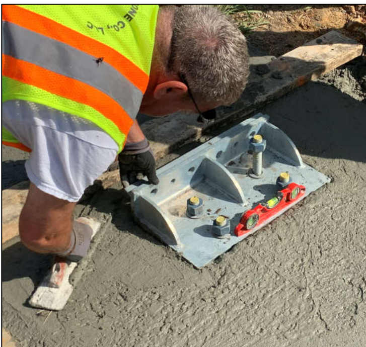
Figure 3: Levelling Anchor Plate
