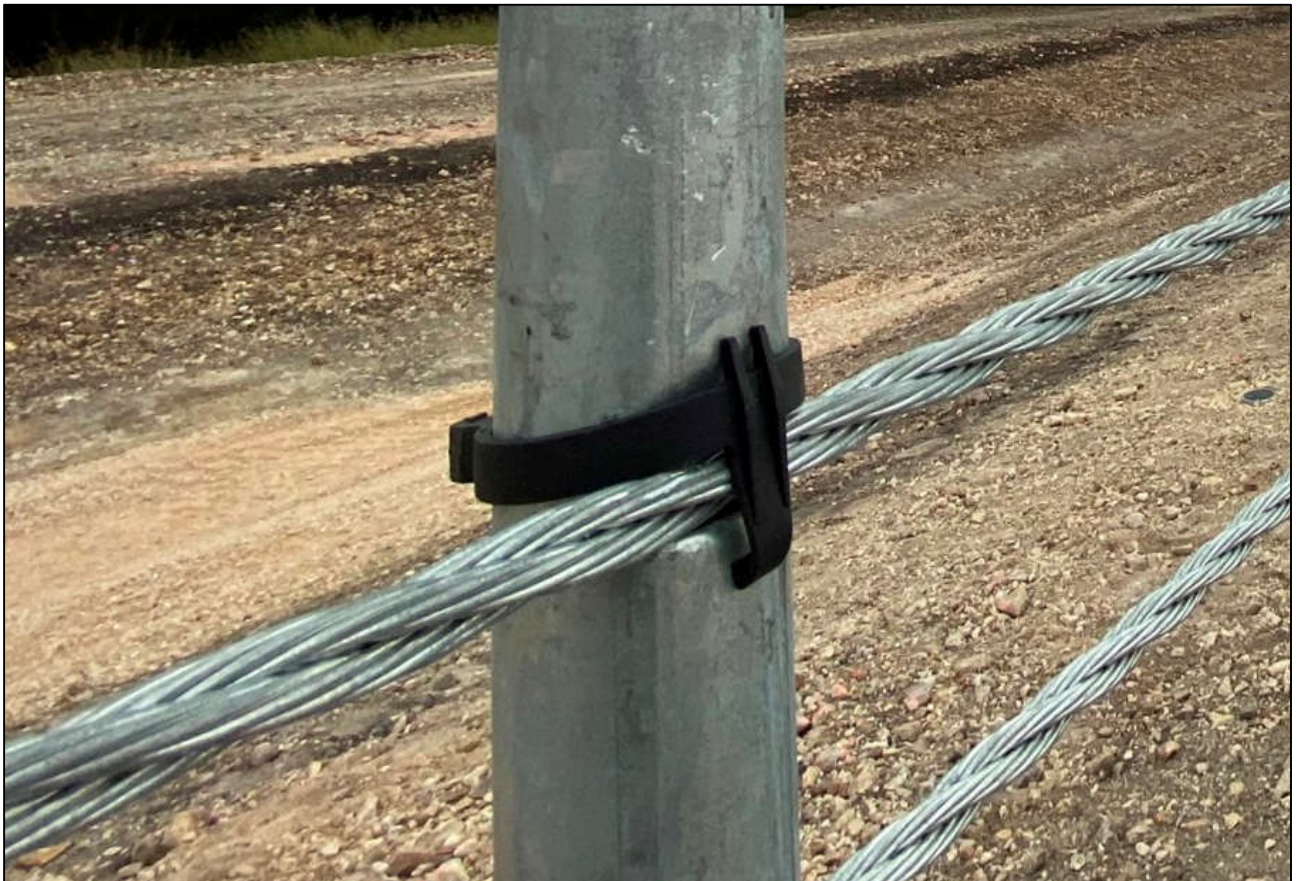
Figure 10: Retainer Clip Position
