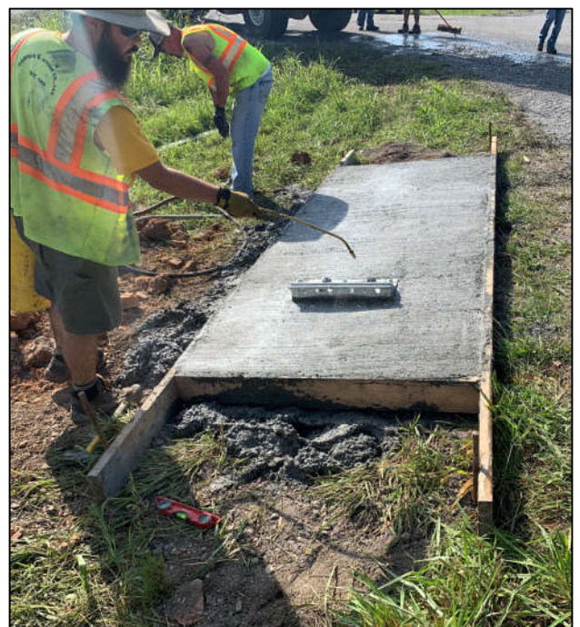
Figure 4: Final Position of Anchor Plate
