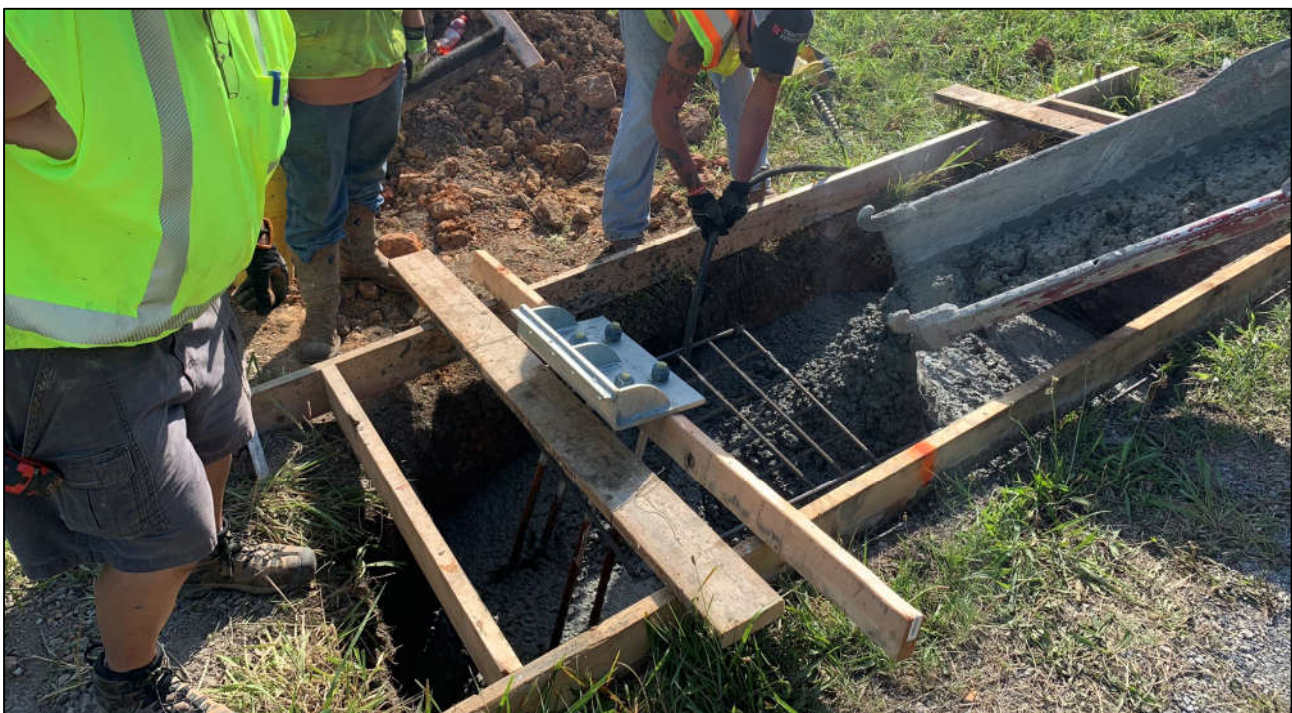
Figure 1: Placement of Anchor Plate
