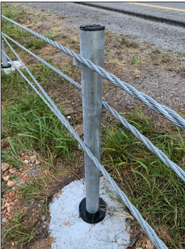
Figure 14: Deflection Post Assembly
