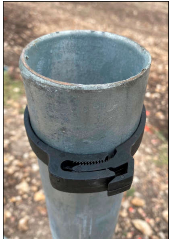
Figure 9: Securing of Retainer Clip
