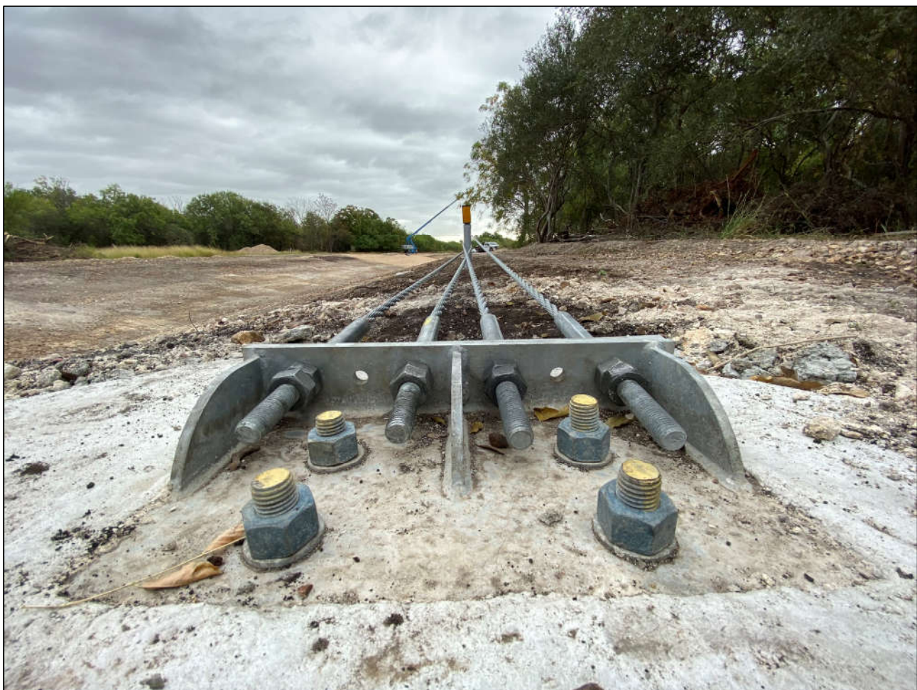
Figure 12: Anchor Bracket Assembly
