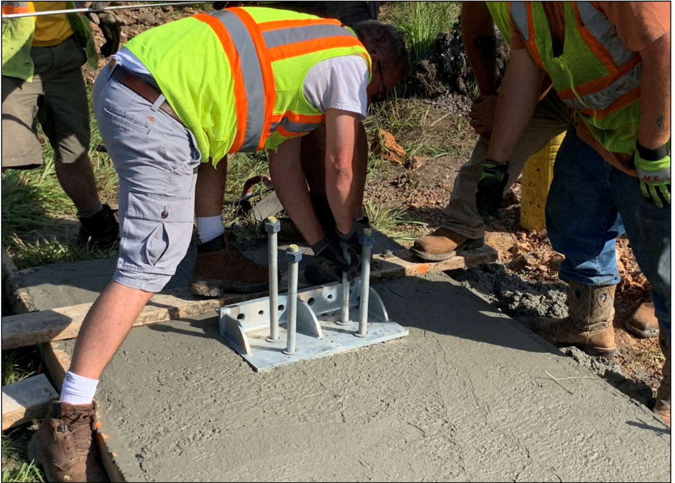
Figure 2: Inserting Anchor Bolts
