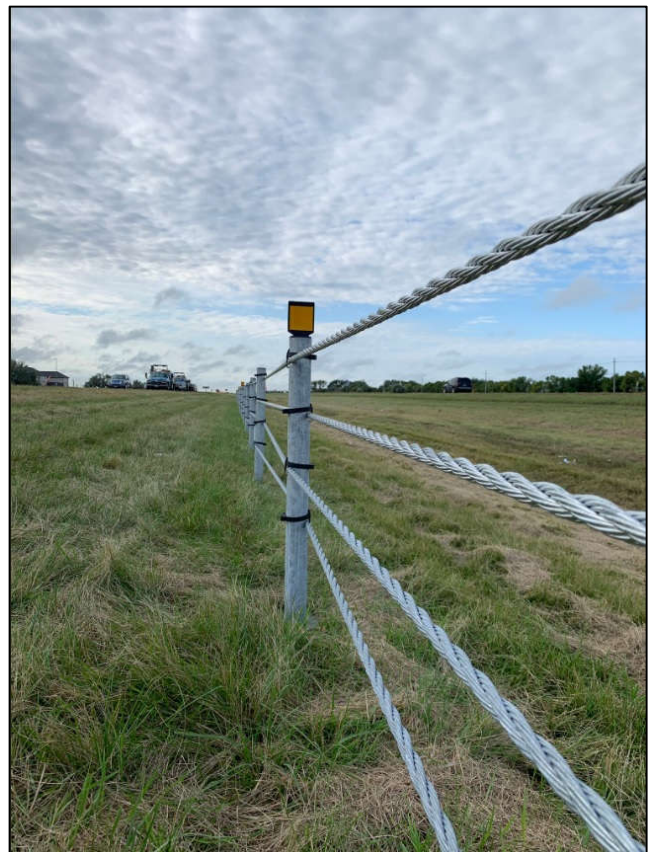
Figure 14: Line Post Assembly
