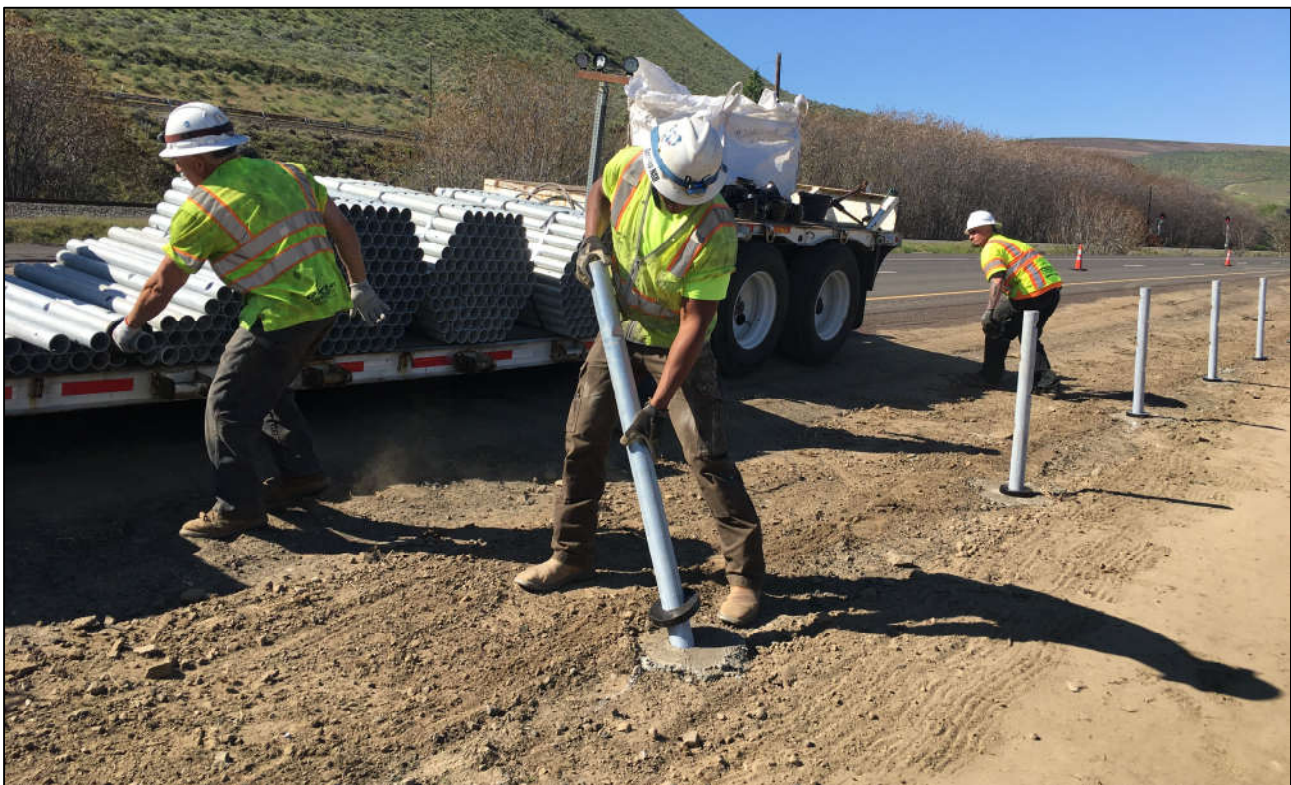
Figure 6: Installation of Line Posts
